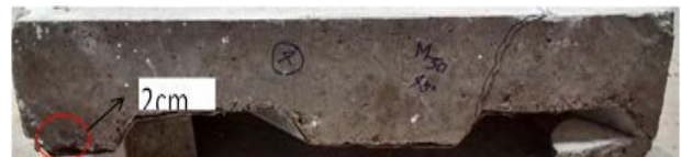
Fig. 13 Slip behaviour for slab 0°
