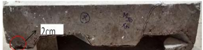
Fig. 12 Slip behaviour for slab 45°
