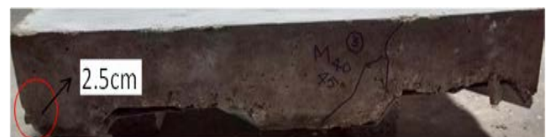
Fig. 16 Slip behaviour for slab 45°
