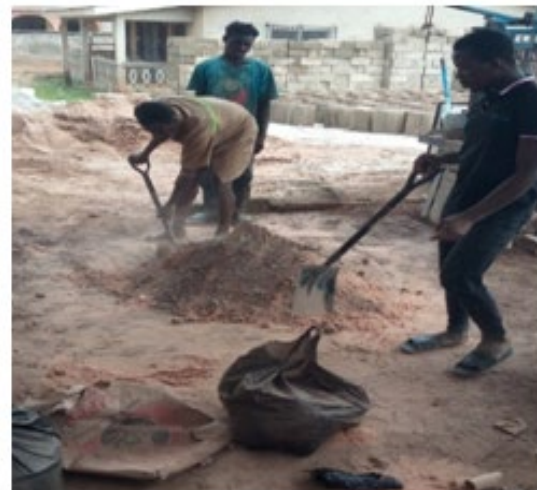
Fig. 2 Mixing of sawdust sandcrete materials
