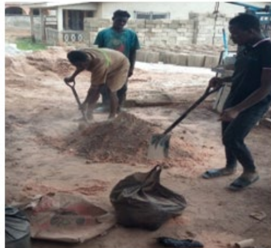
Fig. 2 Mixing of sawdust sandcrete materials
