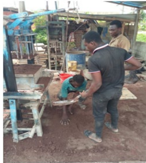
Fig. 4 Mixing of sawdust sandcrete materials
