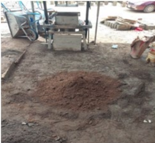
Fig. 1 Batching of materials
