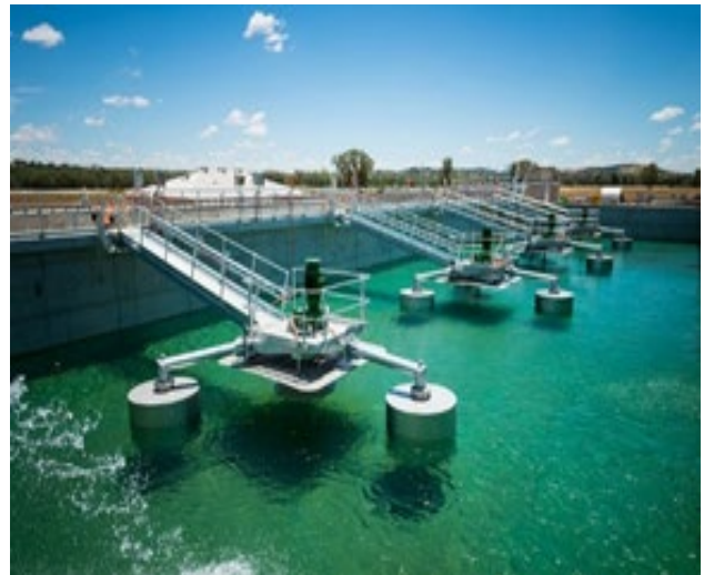
Fig. 8 Chemical removal technique
