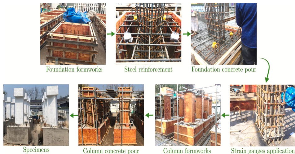
Fig.3 Fabrication sequence for the large-scale Column Specimens: Foundation Formwork, Steel Reinforcement, Foundation Concrete Pour, Column Formwork, Column Concrete Pour, and Finished Specimens Prior to Testing.
